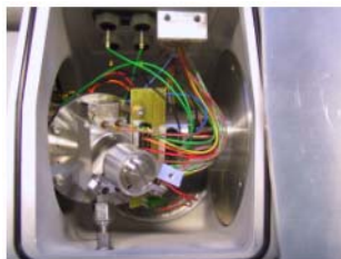
Figure 20 Heater foil cables and nCI body
