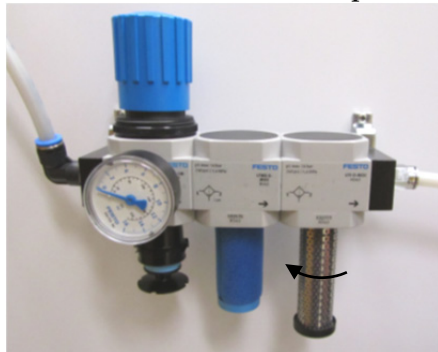
Figure 8. Nitrogen generator gas filters with filter housing removed
