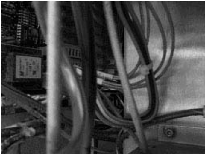
Figure 8 Interior Rear View of GC (Detail)
