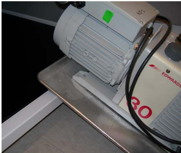
Figure 13 Installing the Dry Pump
