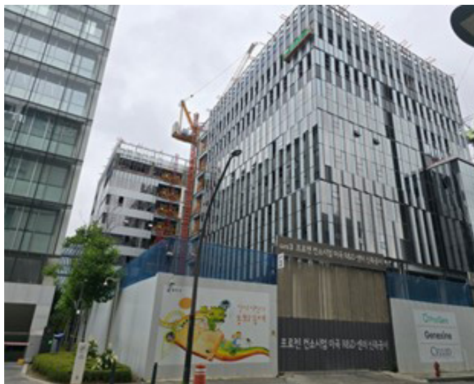
Cellid's new headquarters, under construction in Magok, Seoul, Korea.
